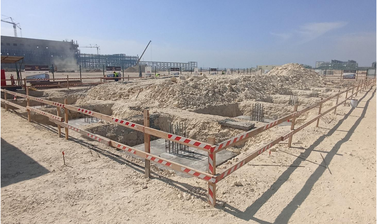
Figure 1: Pilot Plant civil construction works at Jorf Lasfar, Morocco
